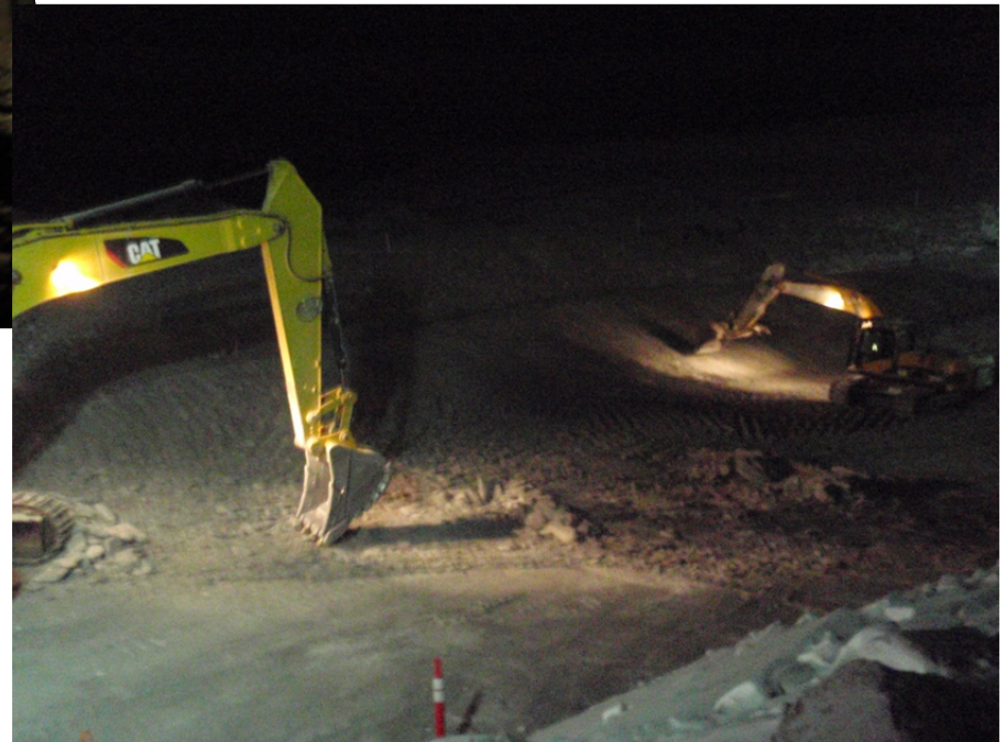
Photo 2: Excavators working on removing frozen 5/8" material in Key Trench, ~ SSW close-up view.
