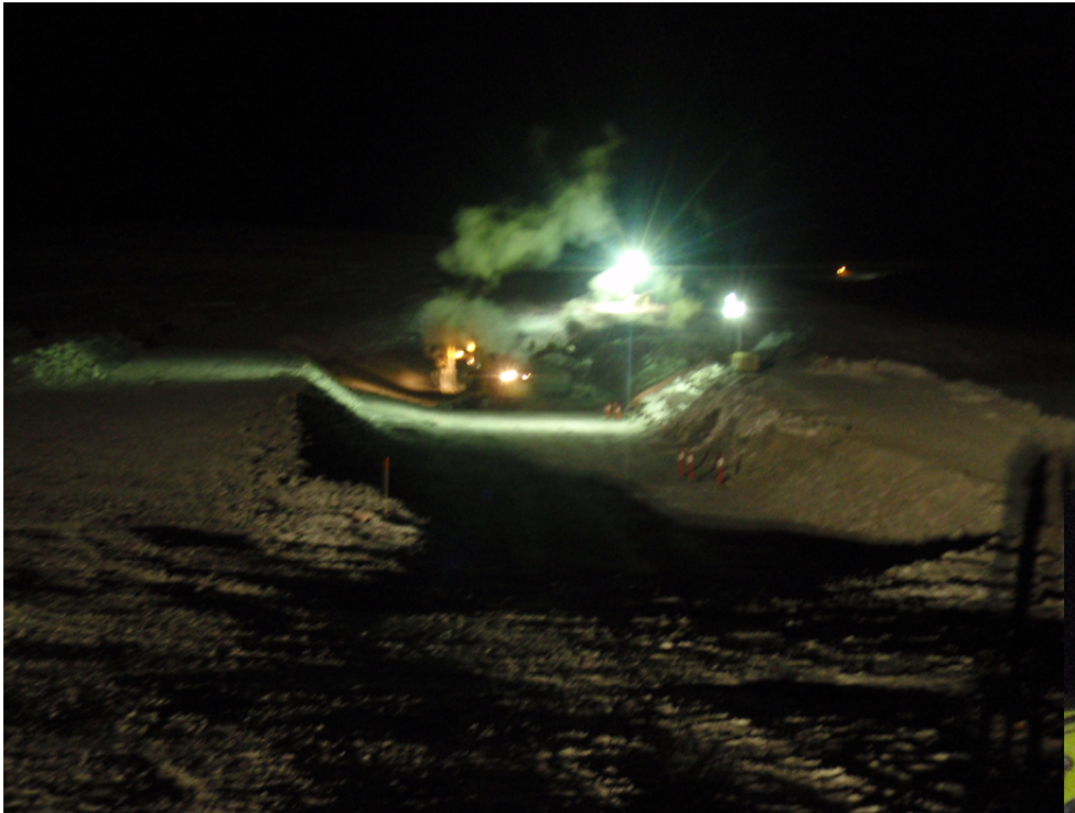
Photo 1: Excavators working on removing frozen 5/8" clear material in North Dam Key Trench, ~ WNW view.
